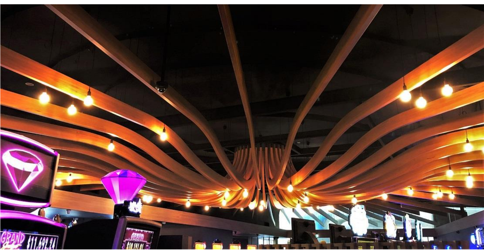
LIONS@Springwood—QLD Architect: Robin Spencer Builder: Mt Cotton Const Product: Ecolite curved ceiling feature in specially toned Blackbutt imagery. The curved shapes were produced in three curved sections. Some of the beams were in lengths of 16 meters and joined using a jig-saw joining method.
