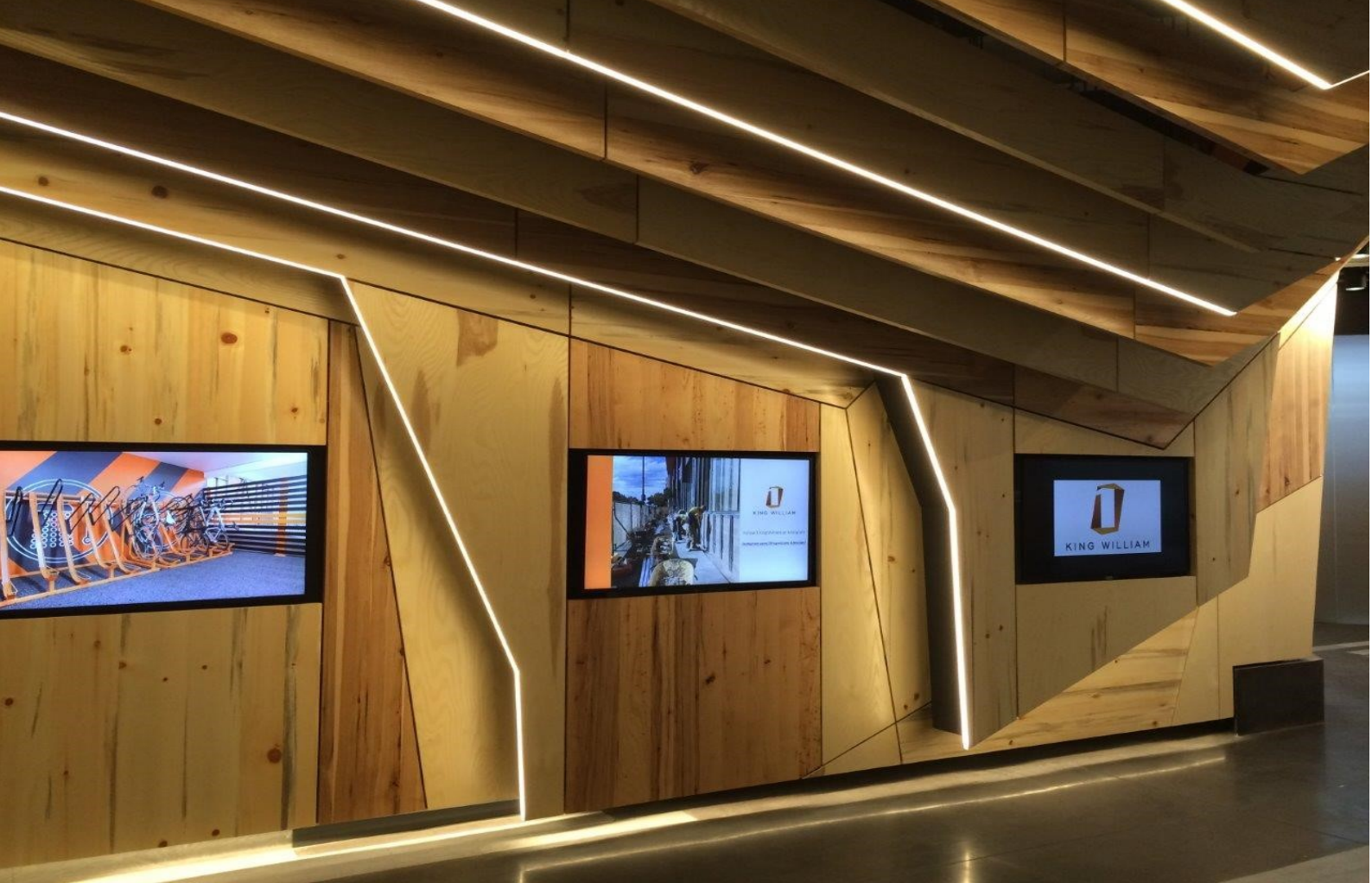
1 King William St, Adelaide Architect: IA Design Joiner: Spry & Spry Product: 35mm thick Ecolite panels with rustic veneer overlay
