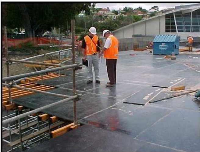
Left – Genuine Structural Formply being used on a construction site
