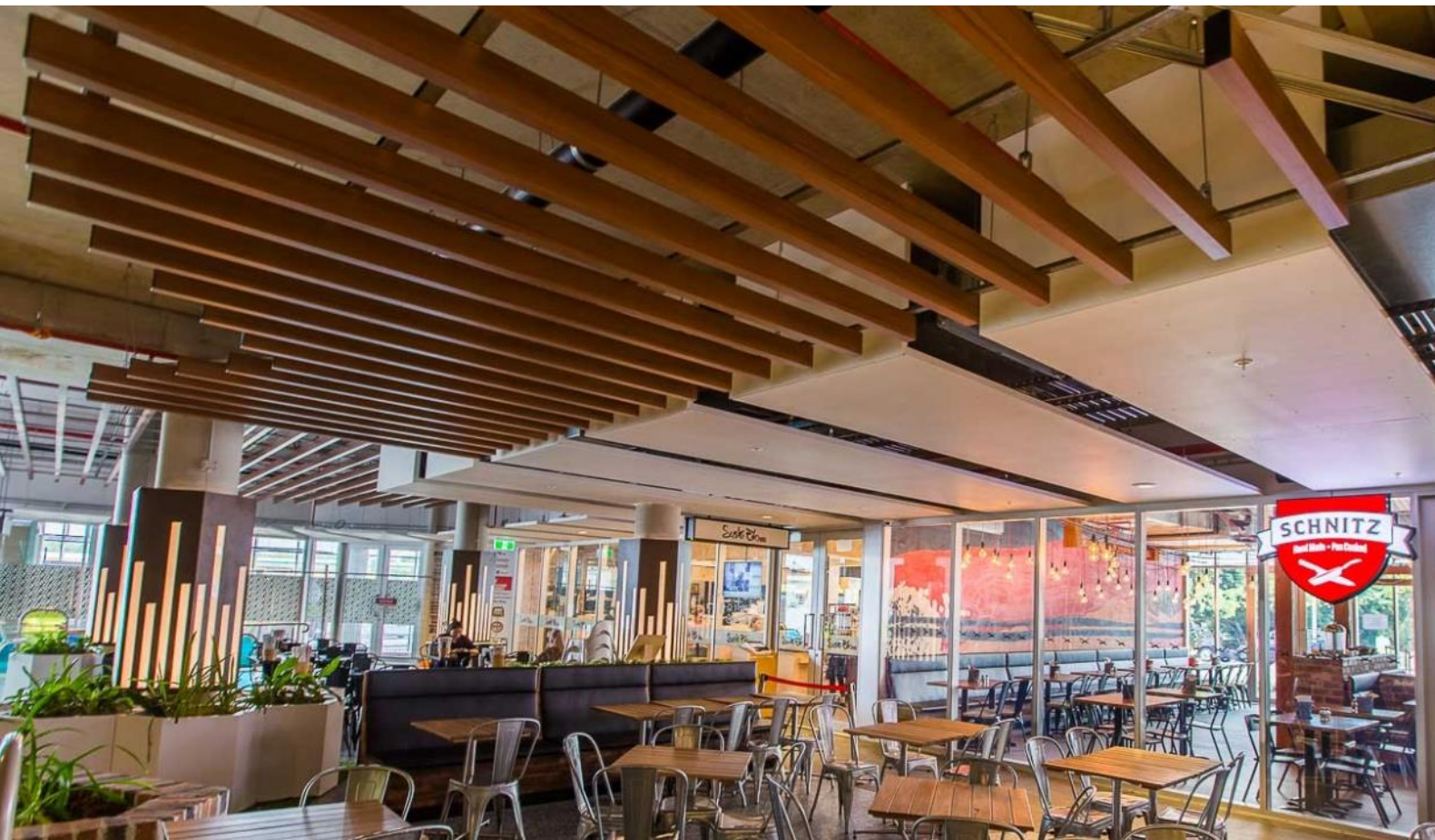
Newmarket Shopping Centre—QLD Builder: Hutchinson Builders Product: FR Aluminium beams with Walnut imagery providing a Non-Combustible solution
