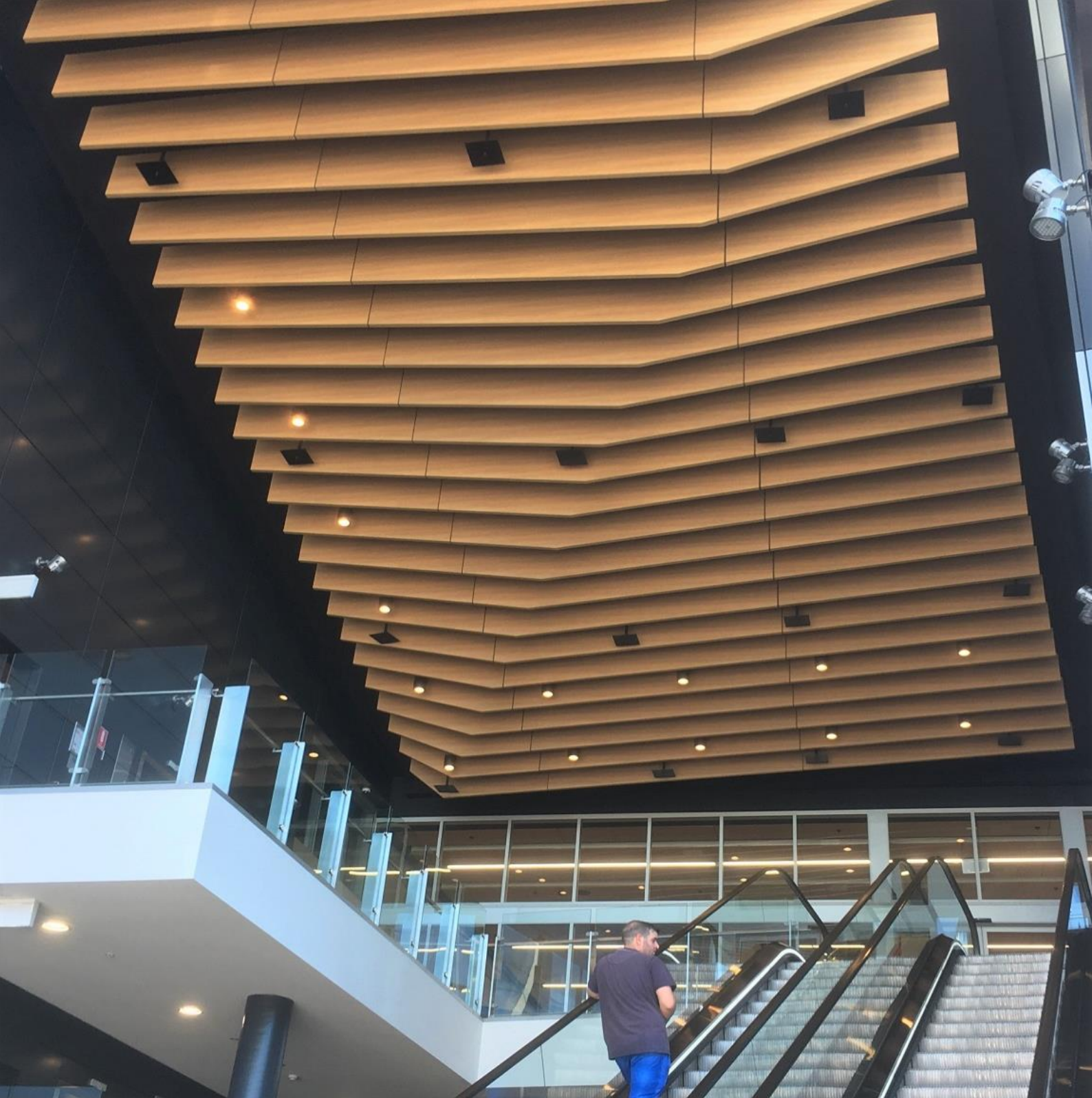
Narellan Town Centre Architect: The Buchan Group Installer: Keystone Linings Product: Ecolite beams faced with Sublime Teak
