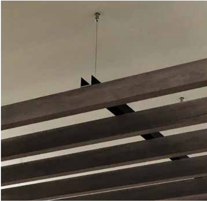
Installation method. Booker Rod and Furring Channel. Beams are top fixed through the furring channel.
