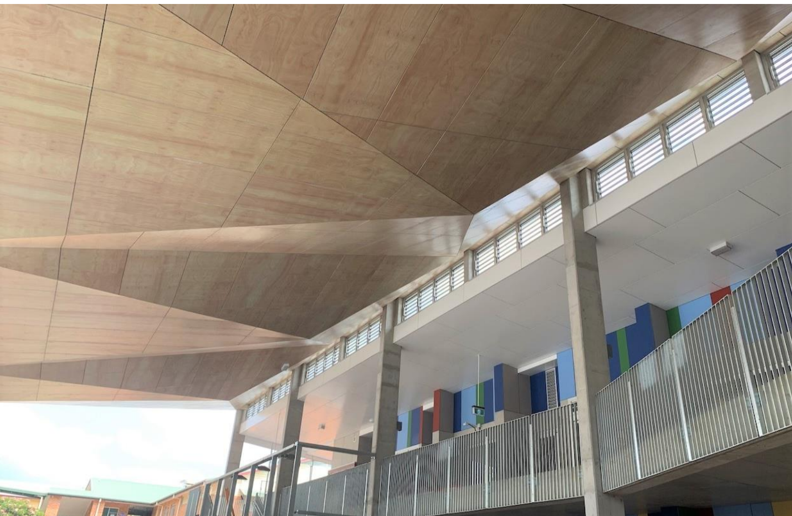
Wauchope Public School—NSW Architect: Conrad Gargett Builder : Lahey Const Installer : Goal Interiors Product : Hoop Pine imagery on FC panels
